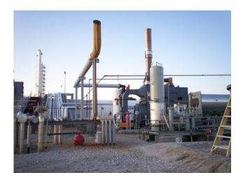
Whether it's being extracted from a newly drilled well (that may have used frac sand) or pumped out a storage field, natural gas requires dehydration or 'sweetening' before it can be introduced into a pipeline. Glycol and amine dehydrators are commonly used for this purpose. No matter what type of reagent is used for dehydration, VOC and organic HAP emissions are generated when the dehydration fluid is recovered in a reboiler.
