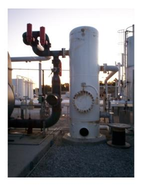
Still, there are challenges associated with designing either the thermal oxidizer or the regenerative thermal oxidizer for service with a dehydrator. The oxidizer must be designed with worst case conditions in mind, not only in terms of VOC loading, but in terms of moisture loading and consideration to the corrosive nature of the vent gas all must be part of the basis of design. Some of the important design considerations are:
