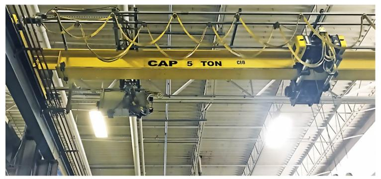
An operator controls the movement of the crane and hoist via push button pendants or radio remote controls. All of these components combined allow the bridge and hoist to move into position over the load. Once the load is lifted, the push button pendant or radio remote control are used to drive the bridge crane to its destination and lower the load.
