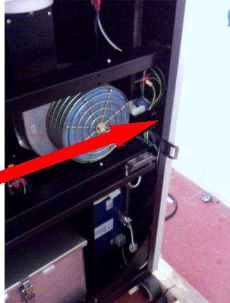
5.2 Measure the voltage supply across the Brown and Blue wires of the input terminal [B] while the contactor is switched on.
