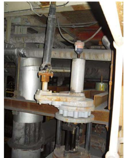
High pressure heater feed outlet with ValvTechnologies' zero-leakage severe service valve installed
