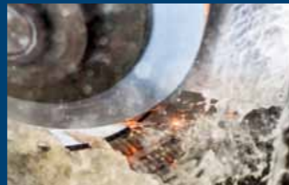
5. Surface Pre-Grinding
