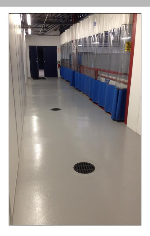
Commercial-grade floor coatings are not considered a do-it-yourself installation and require a minimum of two people. Depending on the formulation, the average pot life of polyurea polyaspartic is only 20 to 30 minutes. The speed and accuracy required is daunting if you have never installed this type of coating before. Get the best results by choosing Pittsburgh Garage to install your polyurea polyaspartic floor coating.
