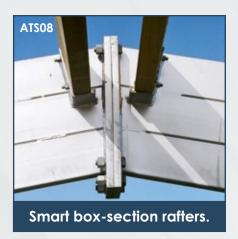
The tough purlin cleats are welded onto the rafters.
