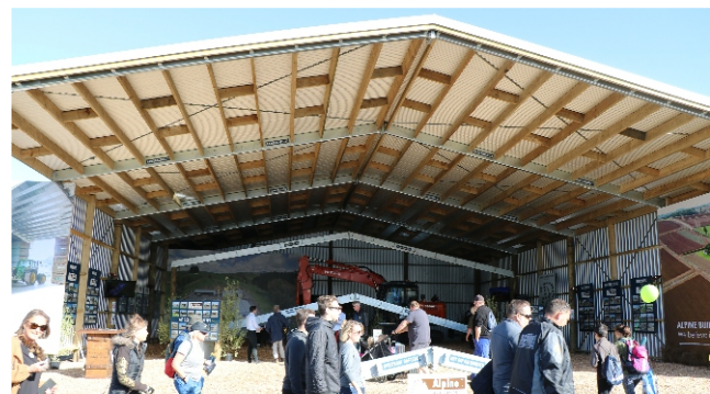
2018: "XXL" 21m clearspan steel rafter launched
