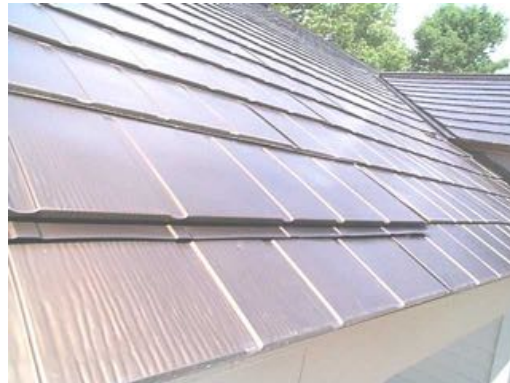
Stored roof shingle placed on top of existing roof
