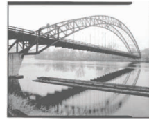
Bellos Falls Arch Bridge
