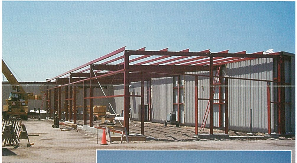
Top photo: Roy's Dodge service center steel erection
