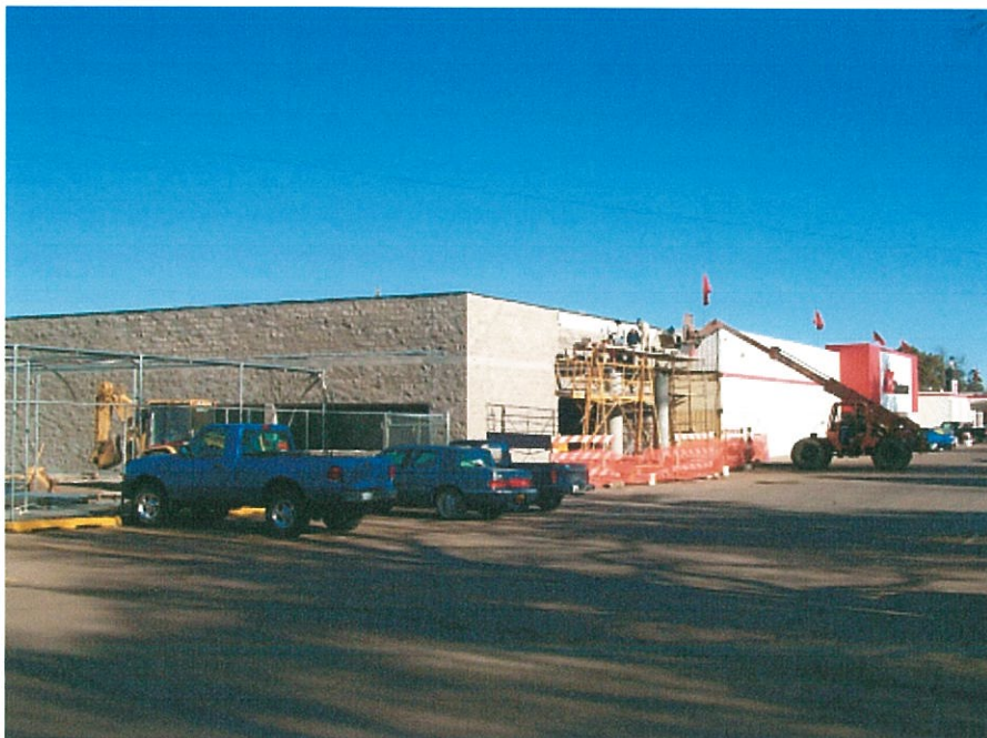
The Ace Hardware addition in progress.
