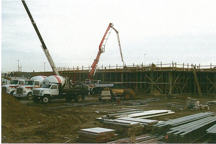
Lacy Construction crews pouring the concrete roof deck for the new surgery addition at St. Francis Medical Center
