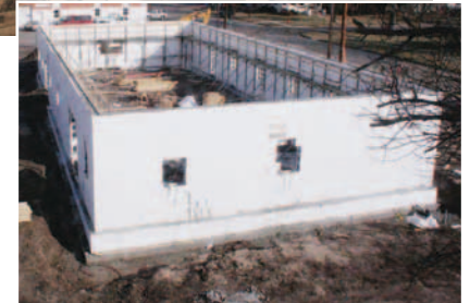
The Archer Credit Union ICF after the concrete was poured.
