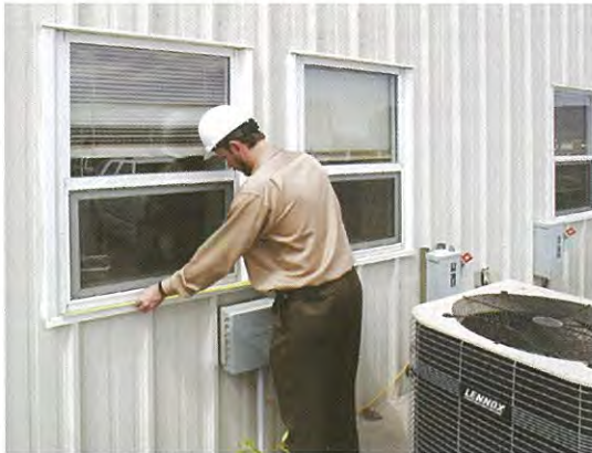
Measuring for a repair estimate.
