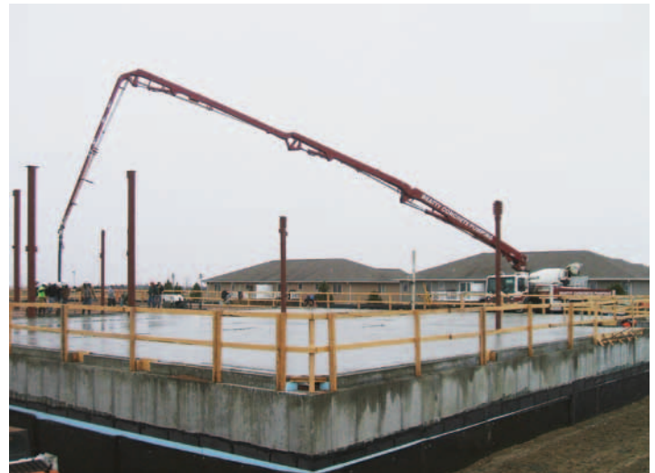
New West floor pour (Try saying that ten times fast!)
