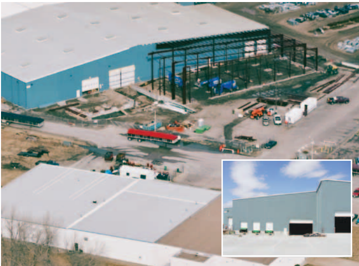
An overhead shot of the MFS expansion. Inset: Exterior view.
