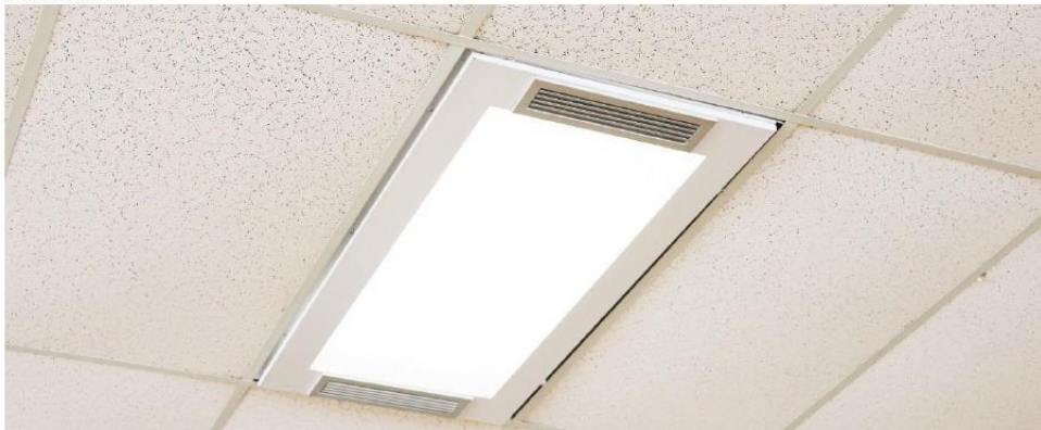
Installed HRMS unit.
