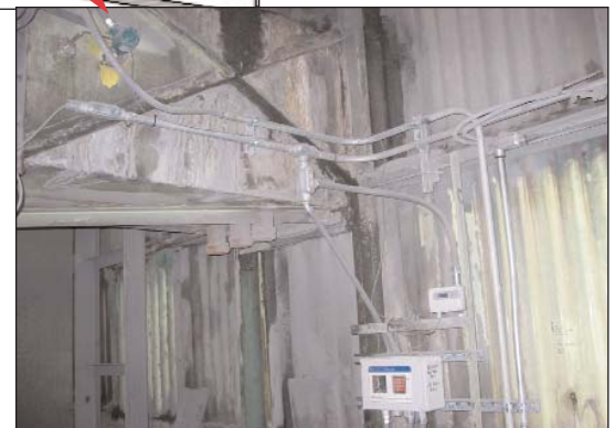
April, 2003 Figure 1 TRIBO.dgd Installed
