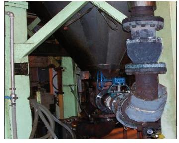
INSTALLATION: A DFT 6" 300# Model Excalibur with severe service Trim was installed vertical flow down for longest service life. Contact DFT for a solution to your problem.
