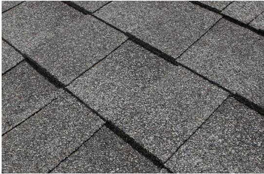
**Asphalt shingles** are the most popular roofing material choice. They're cheap, dependable, and easy to install, and individual shingles can be easily repaired or replaced.
