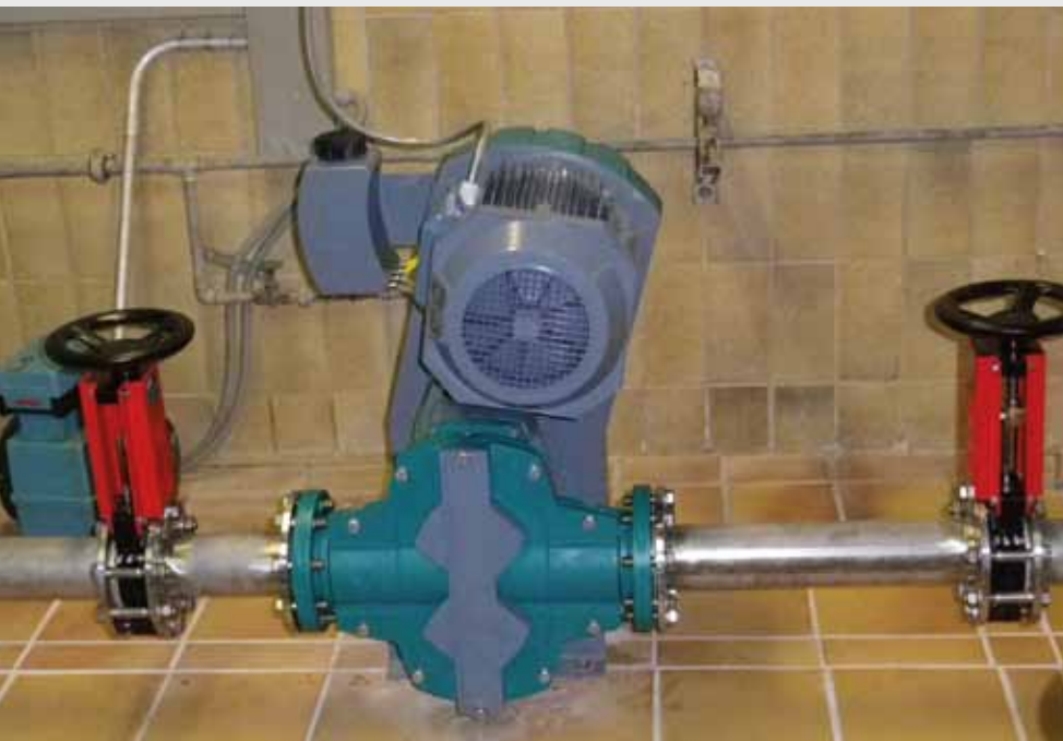
TORNADO T2 pumps sludge in a wastewater treatment plant with 2% solid content at a capacity up to 80 gpm / 18 m 3 /h against a pressure up to 30 psi / 2 bar.
