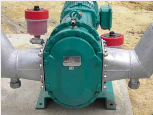
TORNADO T1 used as a feed pump for substrate in a biogas plant with a flowrate up to 175 gpm / 40 m 3 /h at pressures up to 30 psi / 2 bar.
