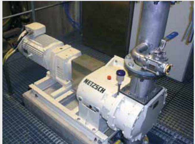
TORNADO T1 in use in a paper mill for unloading kaolin tankers at 330 gpm / 75 m 3 /h against a pressure of up to 60 psi / 4 bar.
