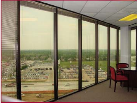
Climate Seal™ Acoustic Series window insert applied over aluminum curtain wall construction for @ Balance America office suites. Houston, TX.
