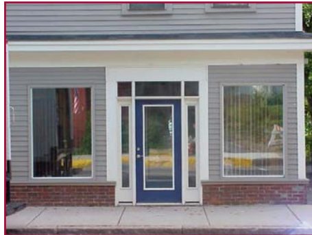
Climate Seal™ Acoustic Series window insert applied over existing storefront glass for maximum sound protection from street traffic. Ipswich, MA.
