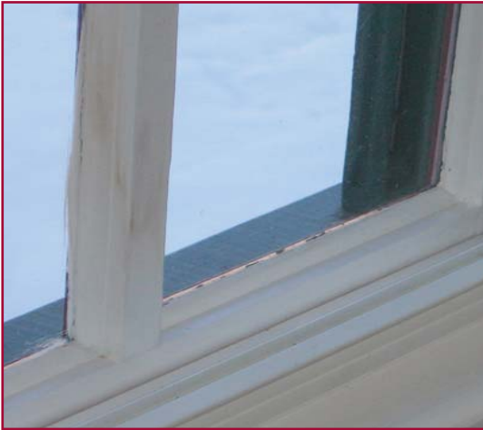
Shown above: WINDOWS INSTALLED – In-Jamb mounting style where the Climate Seal™ window sits inside of the window jamb itself – much closer to the existing window.
