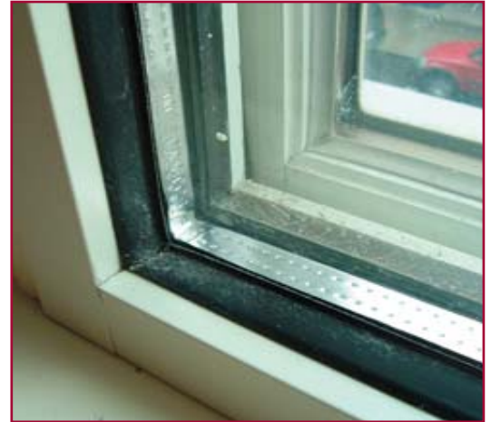
Climate Seal™ Acoustic Series window insert for a residential triple wide double-hung application. Charlotte, NC.
