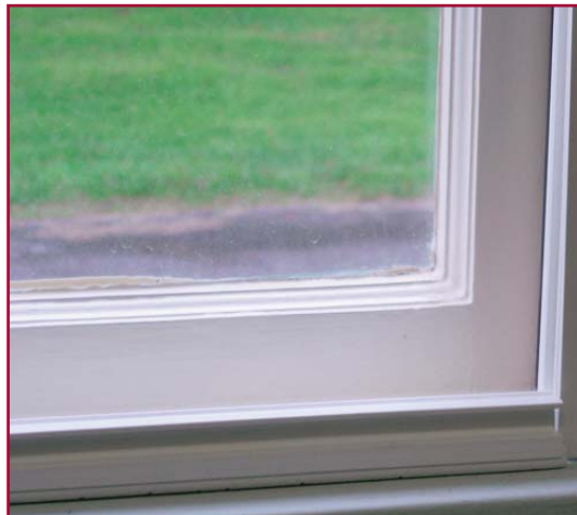
Shown above: WINDOWS INSTALLED – In-Jamb mounting style where the Climate Seal™ window sits inside of the window jamb itself – much closer to the existing window.
