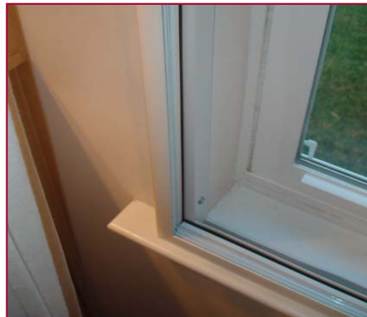
Shown above: FRAME ONLY – Surface mount style installation where the Climate Seal™ window is mounted on the surface of the existing window frame. This mounting style is preferred because of the increased amount of airspace, which allows for maximum sound reduction between the existing
