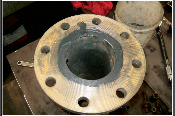
A large dot of Flange Pelseal ® was applied to the damaged area, spread over the spool's face and allowed to cure for 2 hours and a new gasket was put in place.
