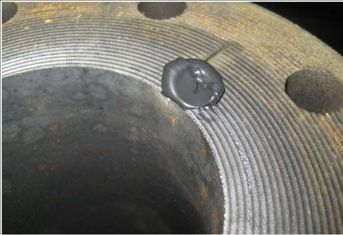
A large dot of Flange Pelseal ® was applied to the damaged area, spread over the spool's face and allowed to cure for 2 hours and a new gasket was put in place.
