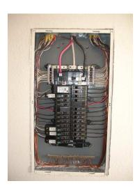
The NEC prohibits the installation of several cables bunched together and run through a knockout or chase nipple.
