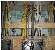
Conductors entering enclosures within the scope of this article shall be protected from abrasion and shall comply with 312.5(A) through (C).
