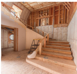
Batts & Loose fill combos are common
