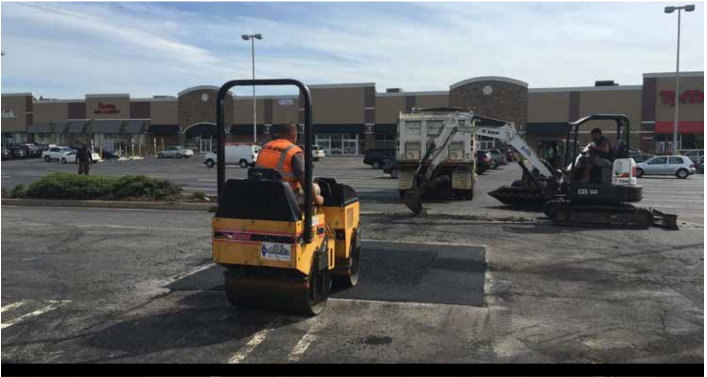
Although Brahney Paving and 1-877-FIX-ASPHALT work on a variety of large projects, they also complete smaller pothole repair jobs.
