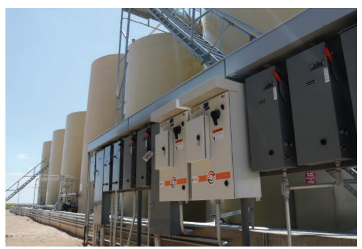
To avoid flaring, vapors in oil storage tanks are often recovered using gas compressors. Compressors controlled by variable-speed drives can result in improved production, higher efficiency and reduced energy costs.
