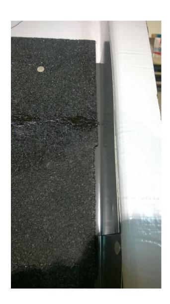
It is good practice to leave ¼" gap between shingles and step flashing. It will allow water to drain and prevent any build up
