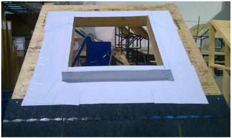
First apply ice & water shield to the bottom, followed by the sides and then the top of the wood curb
