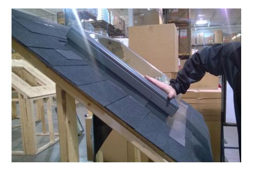
8. Push down on skylight while fastening to curb, using provided fasteners
