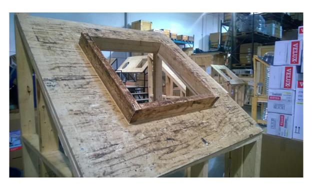
1. Construct a curb with dimensions of 2x4, 2x6 or 2x8. (2x8 Used with tile flashing)
