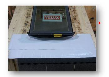
3- Ice & water shield on roof deck prior to overlap on shingle (minimum 3 shingles below)
