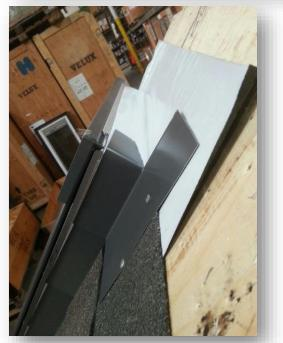
10- Make sure step flashing does not poke a hole in ice & water shield. Recommended to cut on a slight angle
