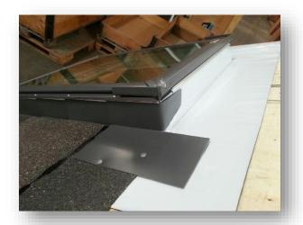
9- Position of last step flashing before top pan is applied
