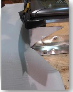
2- Ice & water shield cut on 45 degree angles
