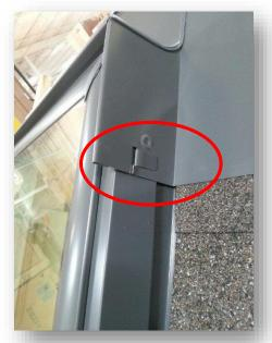
11- Secure cladding to top pan with folded tab
