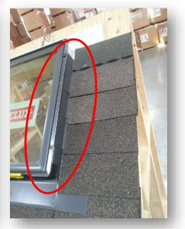
8- Step flashing must be interweaved between each shingle
