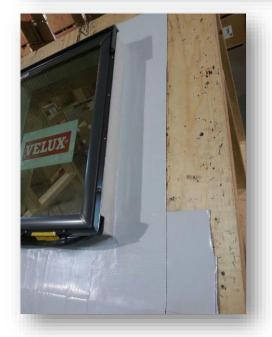
4- All four sides must be wrapped with ice & water shield prior to shingles and step flashing
