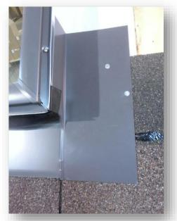
7- Install bottom pan and position UF gasket as in step 5
