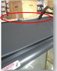
12- Tap down lip on top of head flashing pan
