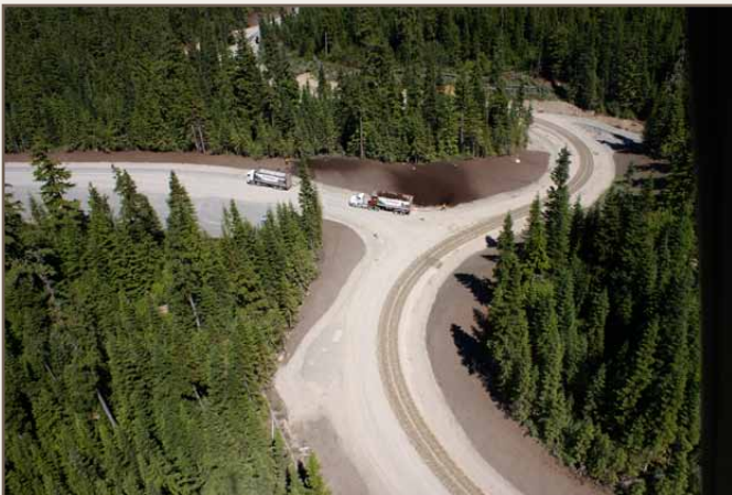
Pneumatic installation and Terraseeding™ of EcoBlanket® for erosion control on soil slopes throughout venue
