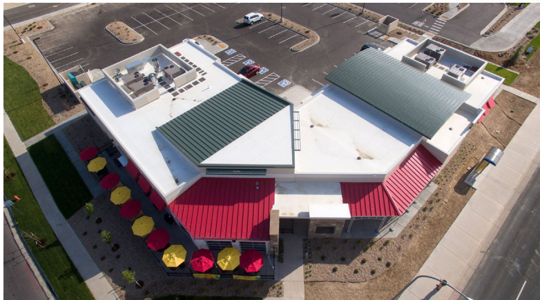
Commercial metal roofing project
