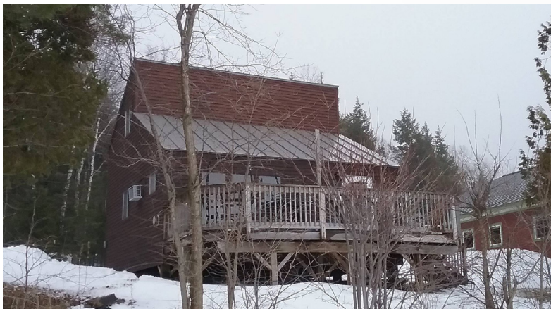
Residential metal roofing project
