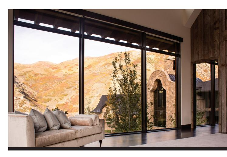
MARVIN SIGNATURE FEATURES: expansive, vertically stacked windows with reinforced steel mulls to support wind and structural load with radius top (left) / large direct set units, mulled with flat steel, to maximize view (above)
