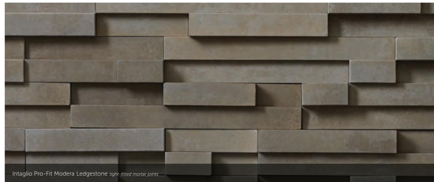
Intaglio Pro-Fit Modera Ledgestone *tight-fitted mortar joints*
