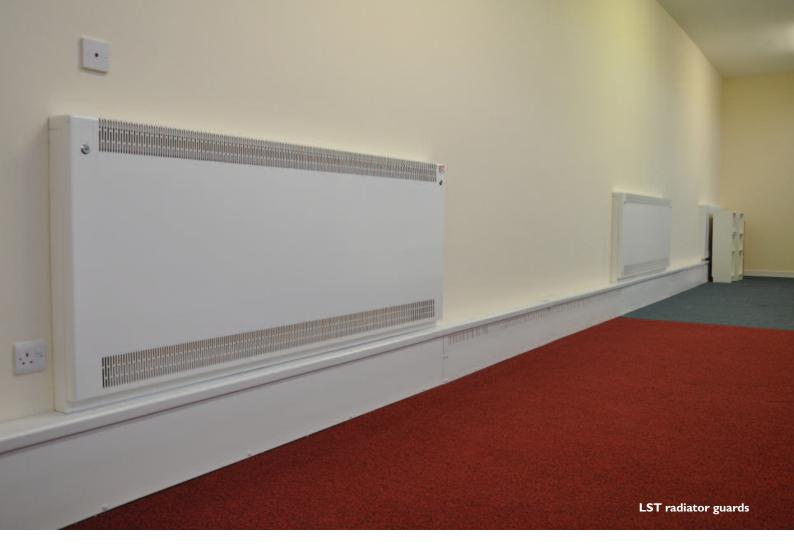
As part of a major refurbishment project, Sandon Primary School in Stoke-on-Trent required a safe, low surface temperature radiator guard solution which could be retrofitted to a range of existing emitters and would deliver robust and practical performance.
