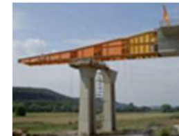
Incremental Launching Method Bridge
