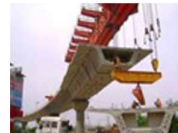
Precast Segmental Method Bridge
