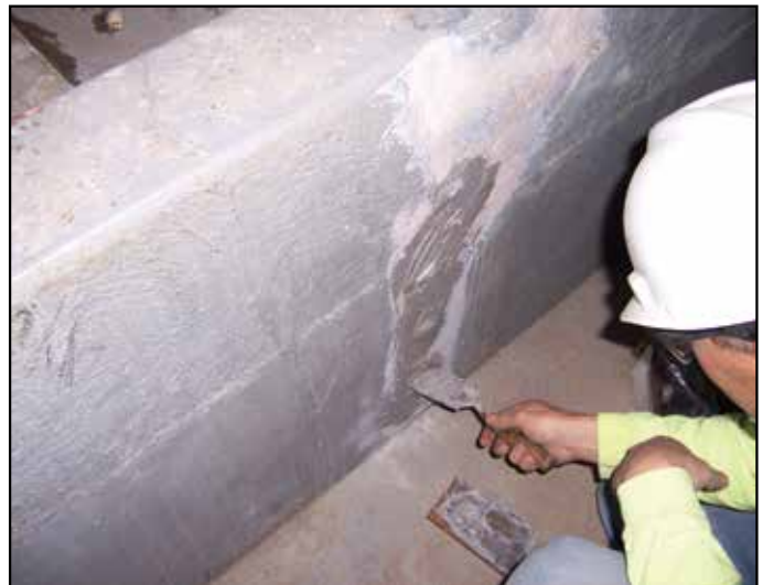
Treating crack with ChemLINE® TSP.
