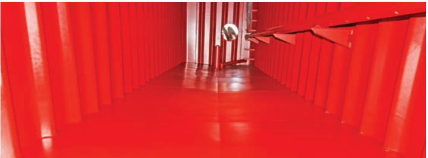
*A tank destined for future HCl storage for Viking Chemicals (top photo), first needs to have the existing dirty greasy epoxy lining blasted and removed, and then chemically cleaned and prepped by MarineLine Turkey at its application facility. (Lower photo) the tank is then lined with two coats of ChemLine® 784/31 delivering a protective solution for storing corrosive Hydrochloric Acid.*
