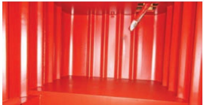
*Up close inspection photos after the final coating shows the very clean, smooth surface that will effectively protect the tank from corrosion against HCl service.*
