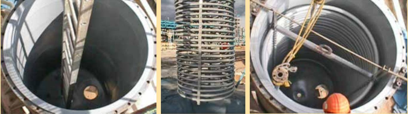
*(Left) Re-lining the R-310 reactor vessel with ChemLine®. (Center) ChemLine® coating of the stainless steel coil used in the reactor. (Right) Reactor and coil, both coated with ChemLine®, ready for service again.*
