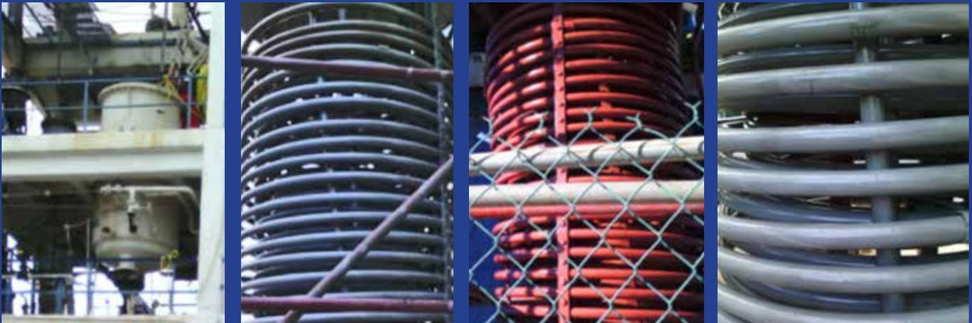
*(Left to Right) Reactor vessel prior to coating in 2014. Stainless steel mixer and stainless steel coil then removed from reactor. Base coat of 'red' ChemLine® 784/32 applied to coil. Top coat of 'grey' ChemLine® 2400/31 applied. (Right) Reactor and coil, both coated with ChemLine®, ready for service again.*
