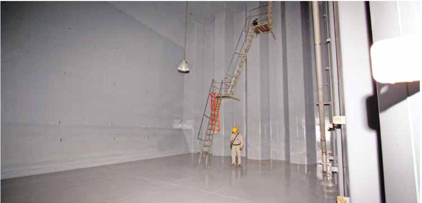
Coating application work is checked by certified MarineLine® inspectors.
