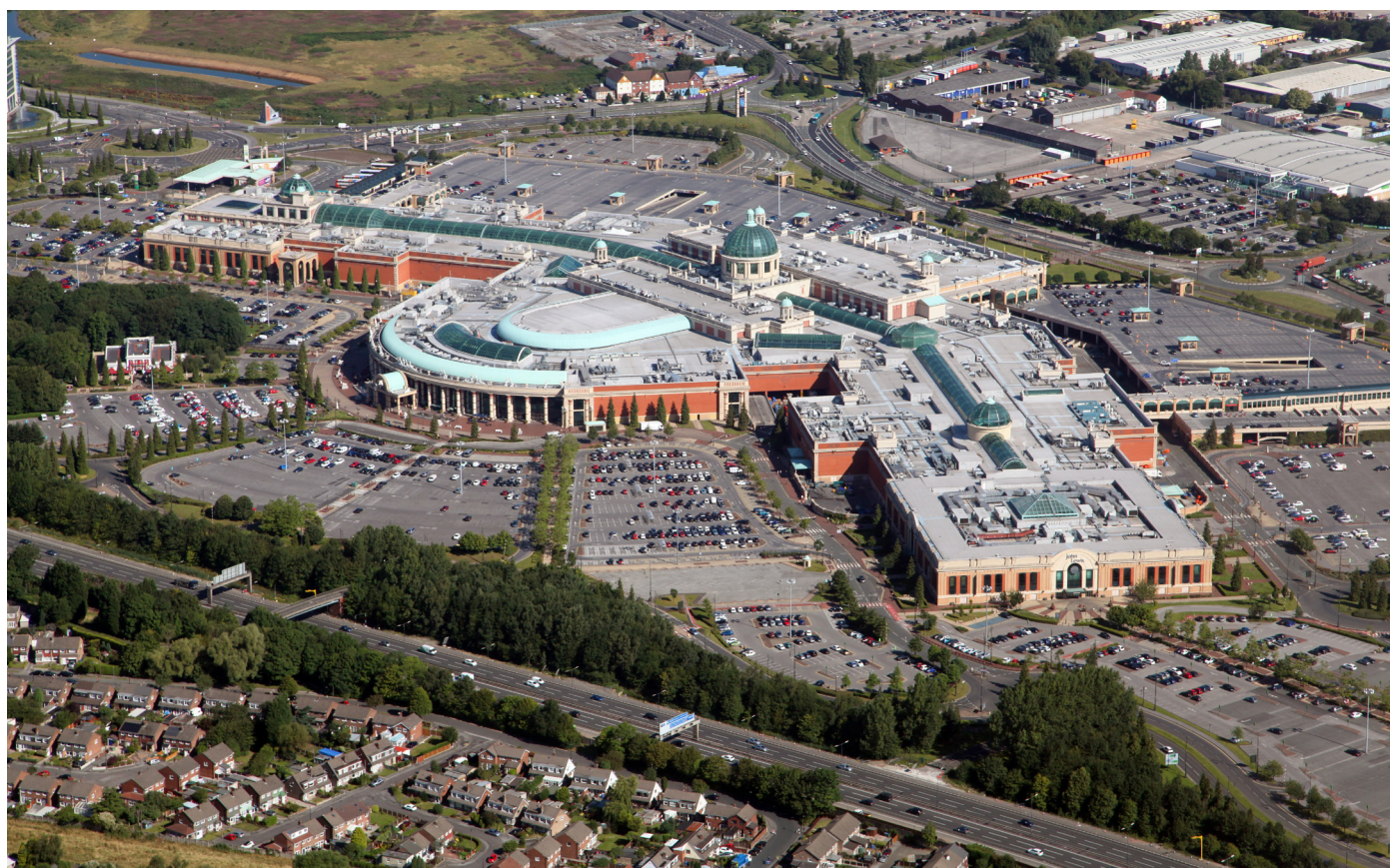
Image 1: Aerial view of The Trafford Centre, Manchester (Photo taken by Neil Mitchell)
