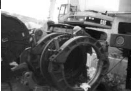
Ken Longfellow and Josh Steward repair a 36" HDPE pipe for International Paper in Jay, Maine.
