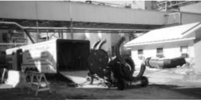
Ken Longfellow and Josh Steward repair a 36" HDPE pipe for International Paper in Jay, Maine.
