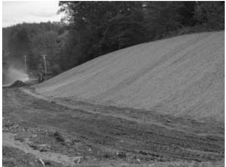
The finished installation in Arcade, NY.
