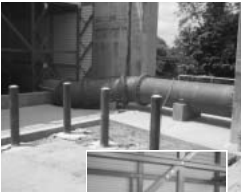
30" flanges and filler pieces installed at Indiana University
