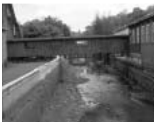
Thomas Hodgson Mill depends on water main for fire protection
