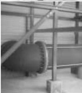
30" flanges and filler pieces installed at Indiana University
