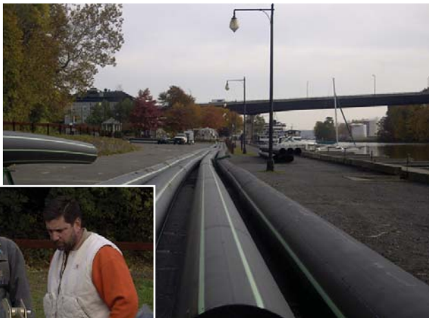
EJP's Joshua Steward and Merritt's Bernie Magee fuse pipe for the Rondout Interceptor-Inverted Siphon Project in Saugerties, NY.
