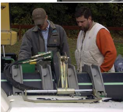
EJP's Joshua Steward and Merritt's Bernie Magee fuse pipe for the Rondout Interceptor-Inverted Siphon Project in Saugerties, NY.
