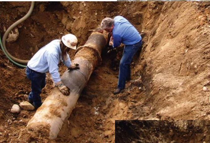
Dramatic scene of the damage and subsequent repairs to a 16" ductile iron water main in the Town of Putnam.
