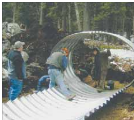
Installing the 30' box culverts.
