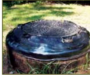
An on site Riser-Wrap training session was conducted in August, 2009, by Ted Tabin of EJP Vernon and vendor Ray McInnis of McInnis Sales. Riser-Wrap seal is a two layer system designed for protection of pipelines and manholes. It seals joints against groundwater infiltration.
