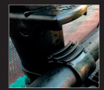
Place the crossover U clip over the Ø90 / 150mm pipe and lock it onto the lower crossover clamp.
