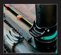
Place the lower crossover clamp around the upright and lock into position using screws.
