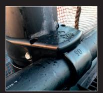
Place the upper crossover clamp around the upright, slide it over the crossover U clip, press upper and lower clamp together and lock the upper crossover clamp into position using screws.
