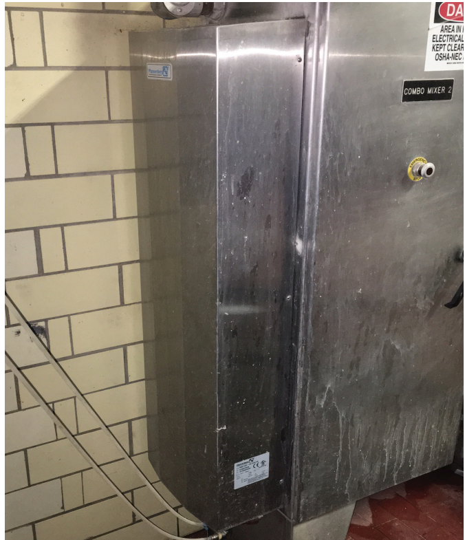
Fig. 4: Pfannenberg's PWS unit installed on enclosure
