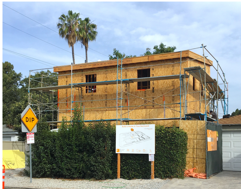
Second Floor Framing
