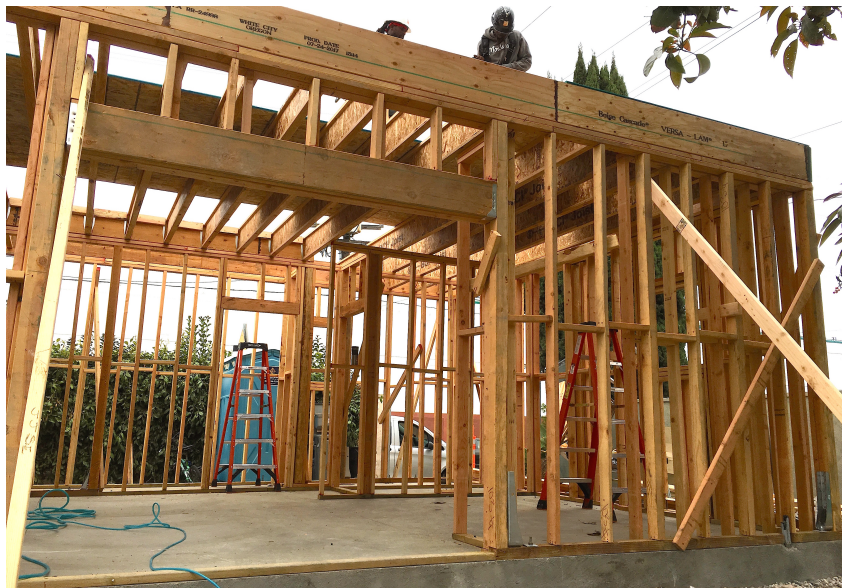
First Floor Framing
