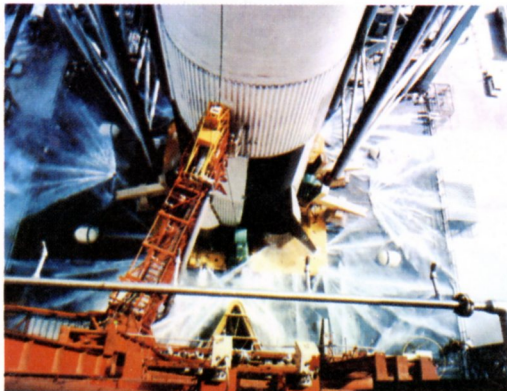
Water Control Systems Provide Fire Protection, Pad Cooling and Quenching
